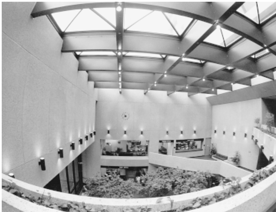
Fig. 3 Why are all these lights turned on? This atrium in a government building is excessively illuminated by a huge skylight. The illumination provided by the light fixtures is not noticeable during the daytime. A single inexpensive photocontrol could save a lot of money and many light bulbs in this area alone.
