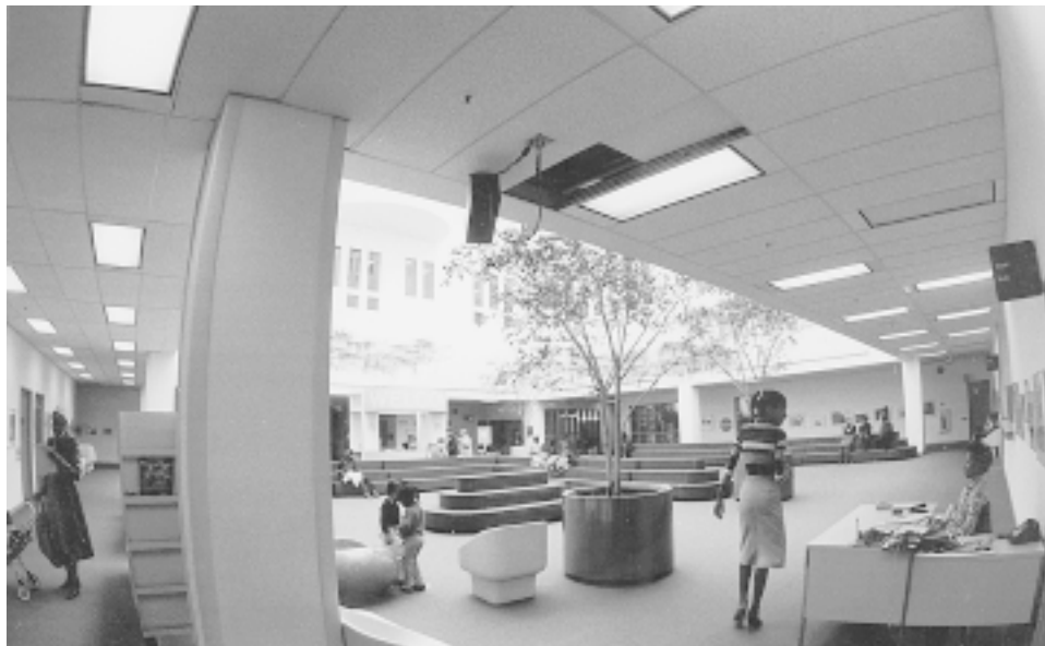
Fig. 4 Area surrounding a large, brightly lit atrium This area deserves several photocontrols. The inner and outer rows of light fixtures should have separate control. And, each side of the atrium should have separate control.
