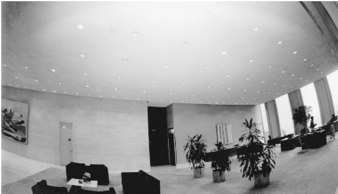
Fig. 2 A good place to retrofit screw-in fluorescent lamps The ceiling of this lobby is a forest of downlights. Screw-in fluorescent lamps provide adequate illumination. Bare lamps provide the best efficiency in the existing reflector fixtures. Their appearance is satisfactory at this distance. Their longer service life greatly reduces the amount of labor required for maintenance.
