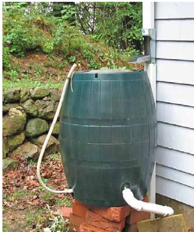
Figure LL-53. A typical rain barrel installation. The adjacent gutter downspout has a diverter that can direct roof drainage into the barrel or can bypass it. This barrel has two bottom outlets, one fixed and one connected to a hose.
