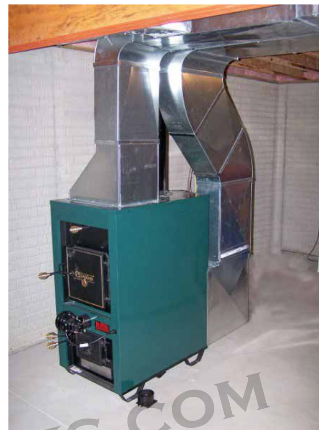
Figure LL-2. A typical wood-fired furnace for a ducted heating system.
