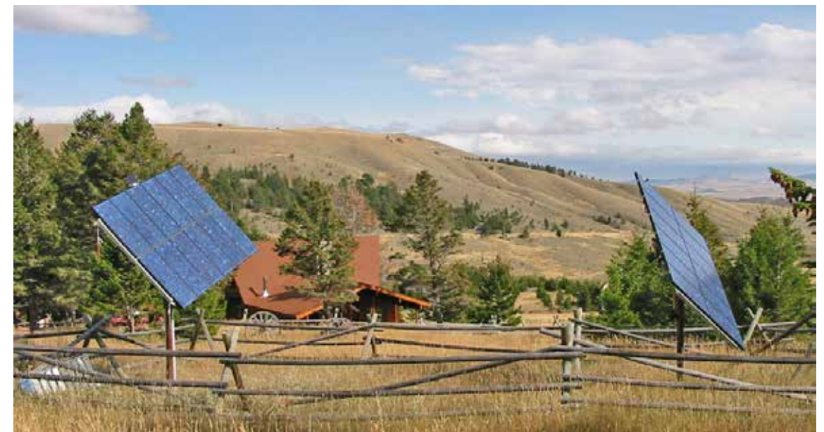
Figure LL-34. The photovoltaic panels for a Wyoming ranch house electrical system. They are installed on mounts that allow them to track the sun.
