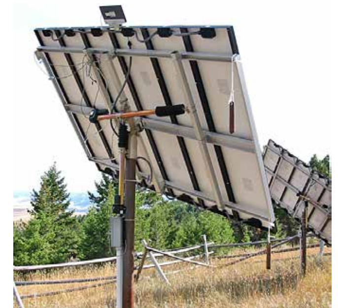
Figure LL-35. The back of a photovoltaic panel, which is thin and light.
