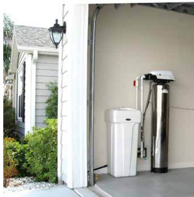
Figure 5-25. Water softener. In the metal cylinder on the right, common salt replaces hardness minerals with sodium compounds. The plastic bin on the left contains salt for replenishing the unit. The sodium that is added to the water may aggravate heart disease.
