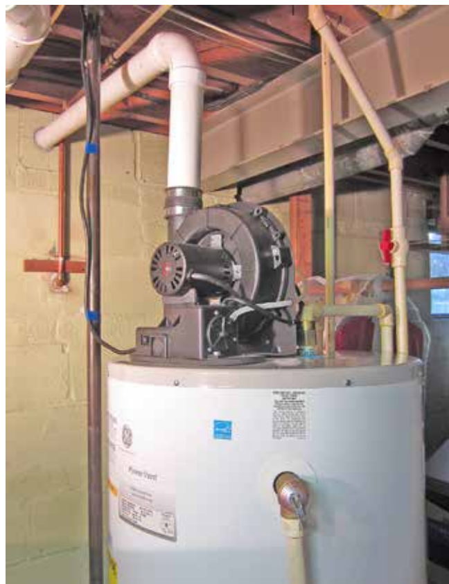
Figure 5-16. A direct-vent water heater. The fan at the top of the heater draws the combustion gas through the heater and discharges it to the outside through a side wall. The exhaust gas is cool enough to be discharged through a plastic pipe.
