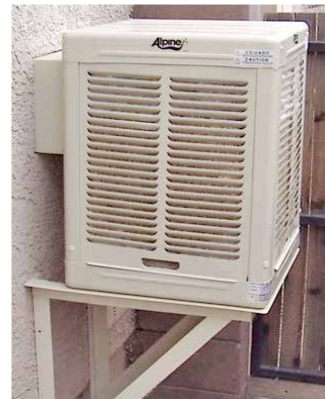
Figure 4-66. Evaporative cooler installed through the wall of a house. This location is superior to the more common roof installation because the entering air is cooler and access for maintenance is easier. Do not install through a window.
