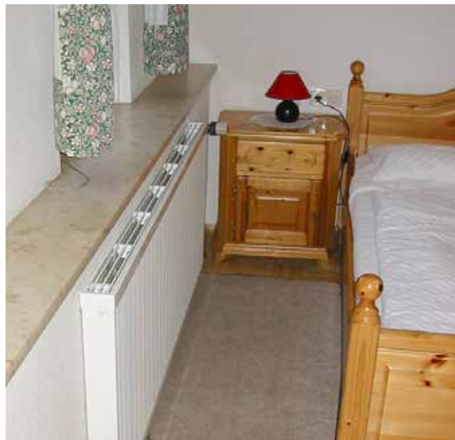
Figure 4-15. Typical hydronic room heater, in Germany. The front face of the unit heats largely by radiation. In addition, the multiple vertical passages provide considerable heating by convection.
