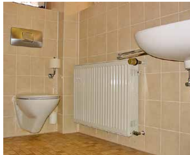
Figure 4-16. Hydronic radiator with a self-contained thermostat, installed in a toilet room in Germany. The heat from the radiator tends to turn off the thermostat, so response is slow and temperature control is crude.
