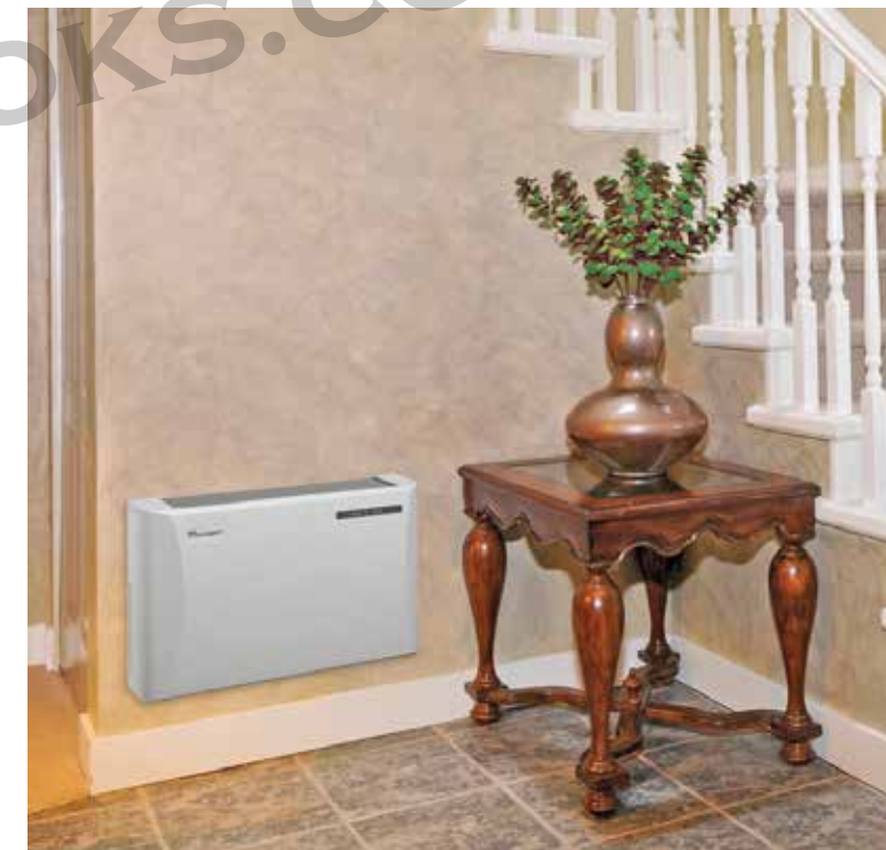
Figure 4-18. An attractive hydronic fan-coil unit.
