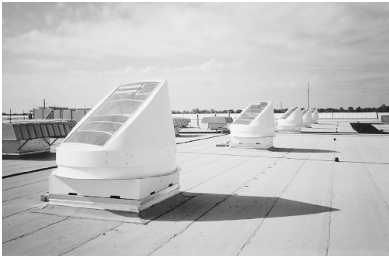
Fig. 14 Sun tracking light pipes The rotating head contains mirrors that reflect direct sunlight straight down the pipe, minimizing losses. However, sun trackers may be less effective than simple light pipes for collecting sunlight from a diffuse sky.
