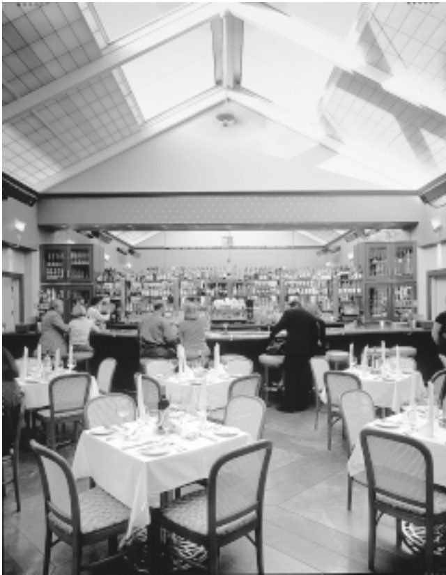
Fig. 4 Adjustable skylight In this restaurant, insulated translucent panels with low light transmission can be retracted to provide a variable amount of skylighting. The layout must keep direct sunlight from entering the occupied area of the space, or diffusion must be used with the skylight glazing.
