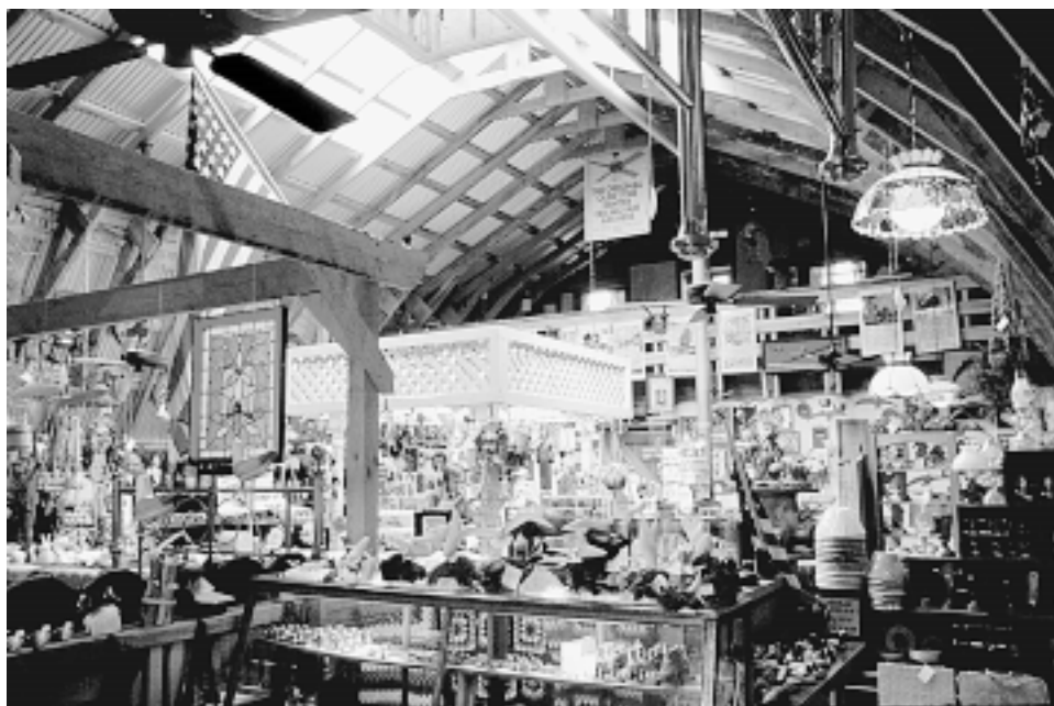
Fig. 3 Skylighting for a variety store The skylight consists of a small area of translucent panels surrounding the cupola. The lighting is effective for the colorful merchandise. The geometry of the skylight does not extend sufficient daylight into the ends of the space, so artificial lighting is needed there. Daylighting of this space was later abandoned, for unknown reasons.
