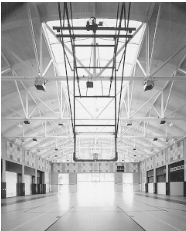
Fig. 7 Gymnasium daylighting with a single large skylight Compare this to Figure 1 of Measure 8.3.2. The barrel roof of this building makes it difficult to install distributed skylights.
