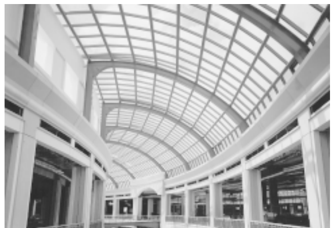
Fig. 2 Large, attractive skylight This is a large amount of glazing area in relation to the illumination requirement.
