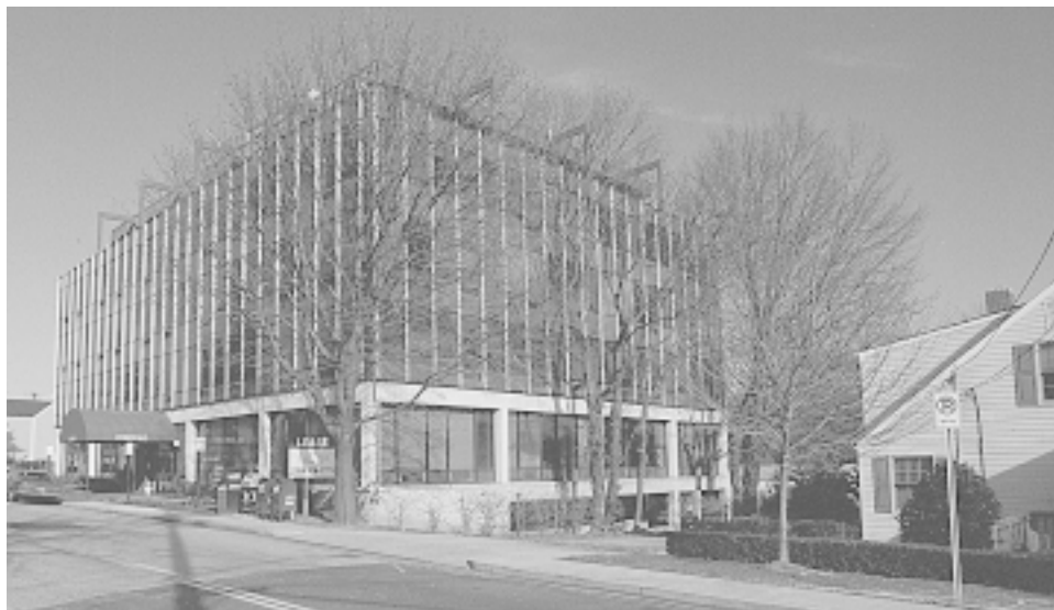
Fig. 1 Tree shading for an office building Above, two trees planted on the south side of this four-story building substantially reduce the cooling load through its large expanses of glass. Below, the trees shed their leaves in winter, allowing the building to benefit from passive solar heating. The trees form an effective visual divider between the office building and other buildings in this mixed-use neighborhood.
