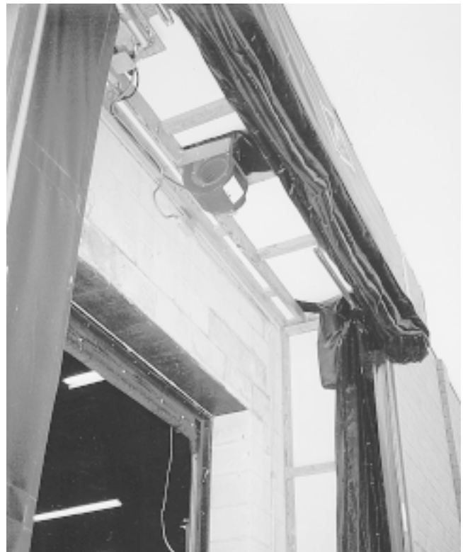
Fig. 4 Inflatable seal deflated The small fan at the top of the unit provides all the pressure that is needed for effective sealing.
