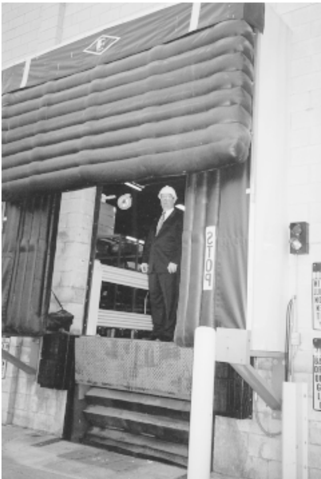
Fig. 3 Inflatable dock seal The upper part of the seal is inflated, the sides are not. Note the guide post, the bumpers to keep the trailer from backing too far into the seal, and the spotlight. Correct alignment is essential for sealing and for protecting the seals.
