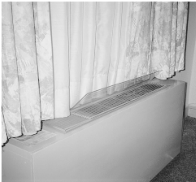
Fig. 3 Simple, effective baffle on a fan-coil unit This piece of flat clear plastic is bent to form a flange that is screwed to the top of the unit. It keeps the unit's air discharge from blowing behind the curtain and being trapped against the window.
