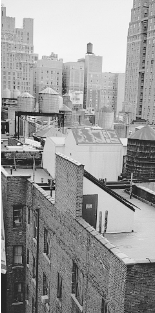
Fig. 2 Gravity tanks These buildings use gravity tanks for two purposes, pressurizing the domestic water system and providing a separate source of water for fire protection. In most of these buildings, separate tanks are used for the two purposes. The elevation of the tanks above the roofs provides adequate pressure for the upper floors.
