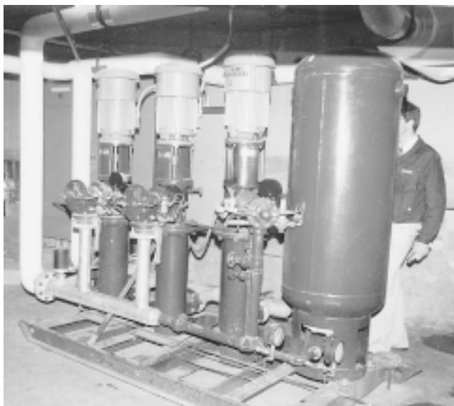
Fig. 4 Service water pressurization equipment in the basement of a tall office building The closed tank on the right maintains constant water pressure. The three pumps on the left operate in sequence.
