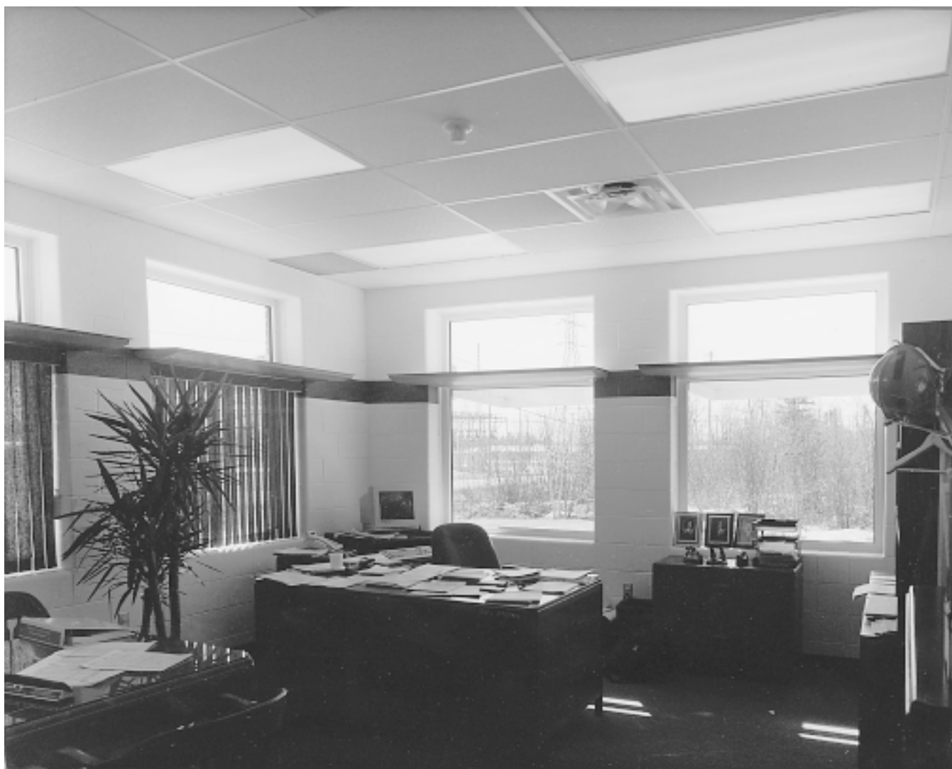
Fig. 1 Light shelves These are installed directly against the windows, just high enough to avoid being a hazard. The top of each shelf is a mirror, and it must be kept clean. Only windows exposed to direct sunlight are eligible. Glare must be avoided from the portion of the window below the shelf. The windows at left have internal shades. The windows at right are shaded by an external fixture, shown in Figure 4.
